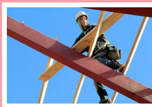
Conecting the Steel6
