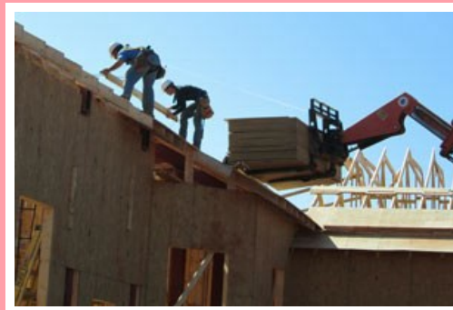
Laying the Roof
