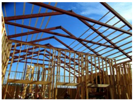
See Through Roof
