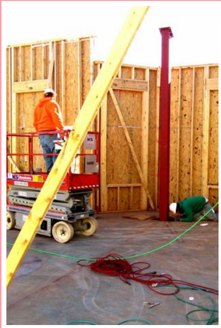
Tightening the Bolts
