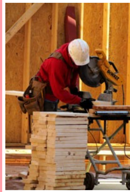
Cutting the Roof Joices
