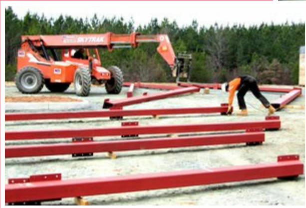
These get Attached to the Columns
