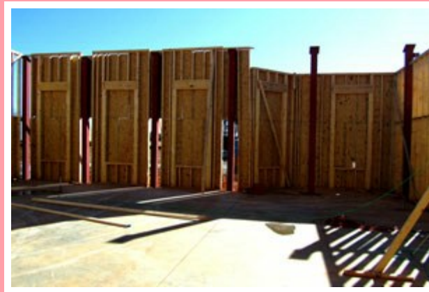
Columns in Place
